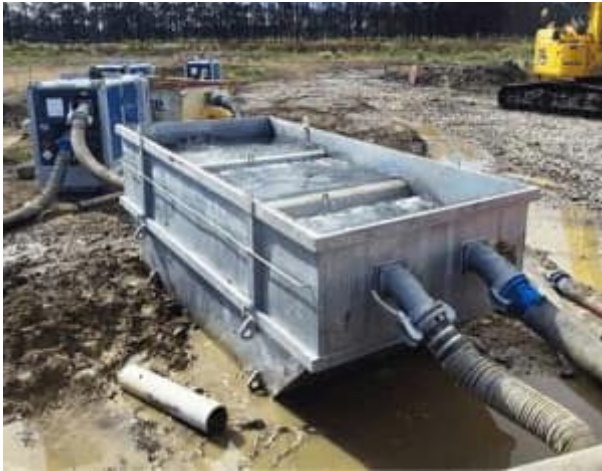
Figure 8: Temporary settling tank set up.
