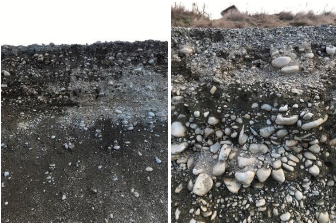
Figure 6: Client Photos from the Quarry Walls
