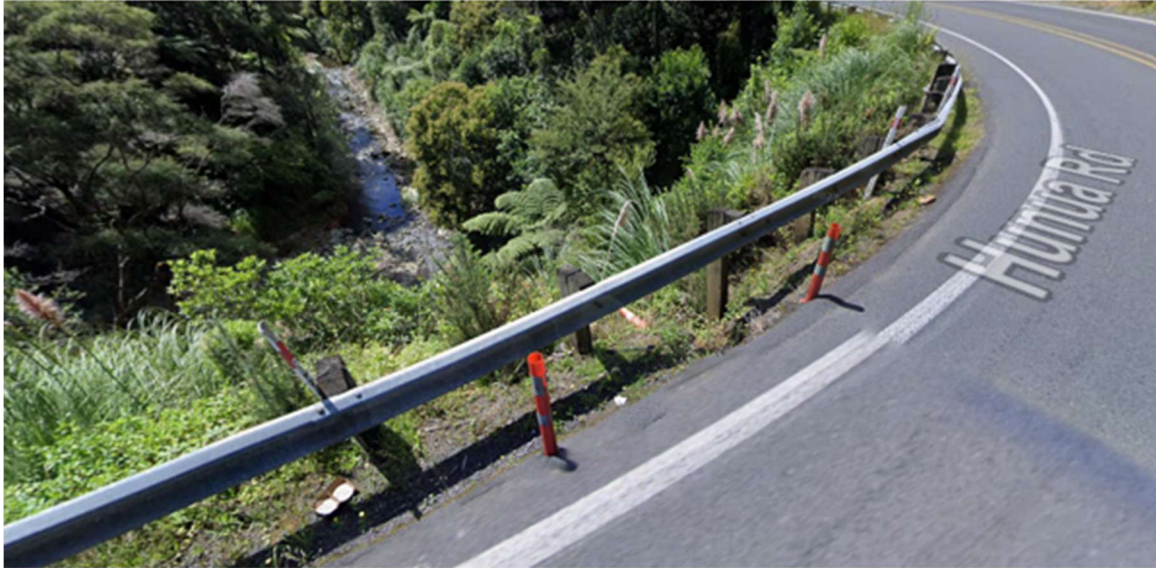
Photo 1: Road safety barrier next to gorge on Hunua Road. Corresponding Commute tracking drawing number 4B.
