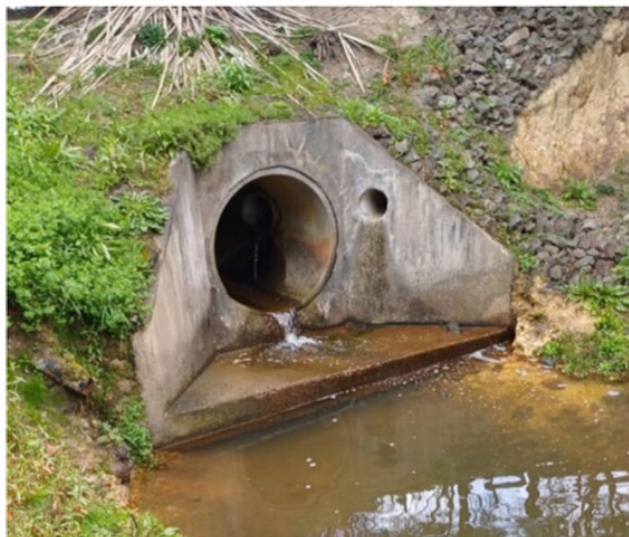
Figure 1 Existing Watercourse 1 outfall from existing 900mm pipe
