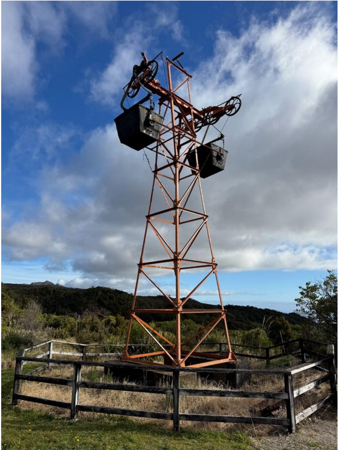
Figure 8. A surviving aerial cableway support tower above the Denniston Brakehead (Feature A39). This tower is maintained by DOC, and the two buckets have been mounted on the tower to give the impression of how it would have appeared when working
