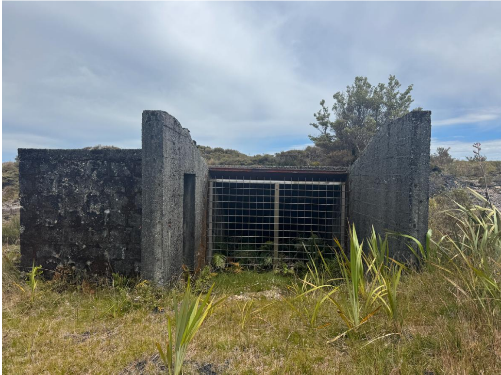
Figure 31. The concrete/brick shell of the Sullivan Mine fan house with the incline tunnel inside (Feature 24)
