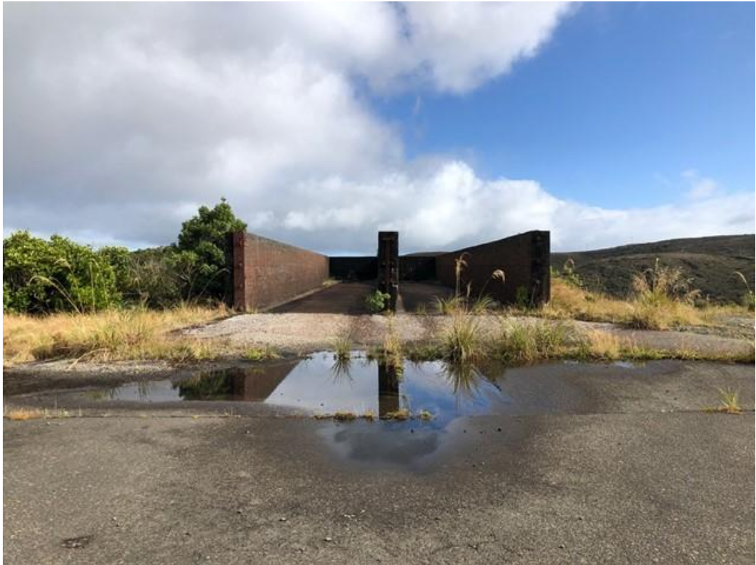
Figure 19. Whareatea dewatering pads (Feature 16) from the lower part of the truck loading apron
