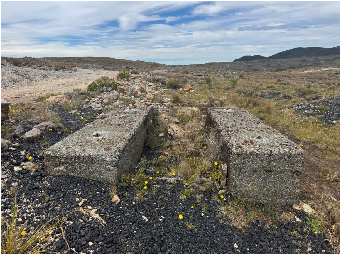
Figure 9. Double support tower foundation for the aerial cableway near Sullivan Mine (Feature A13)
