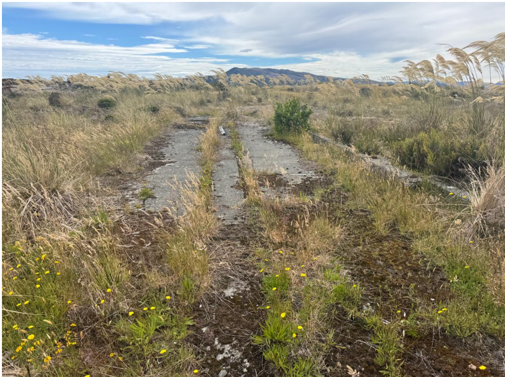
Figure 32. The concrete foundation of the workshop/store at Sullivan Mine (Feature 32)
