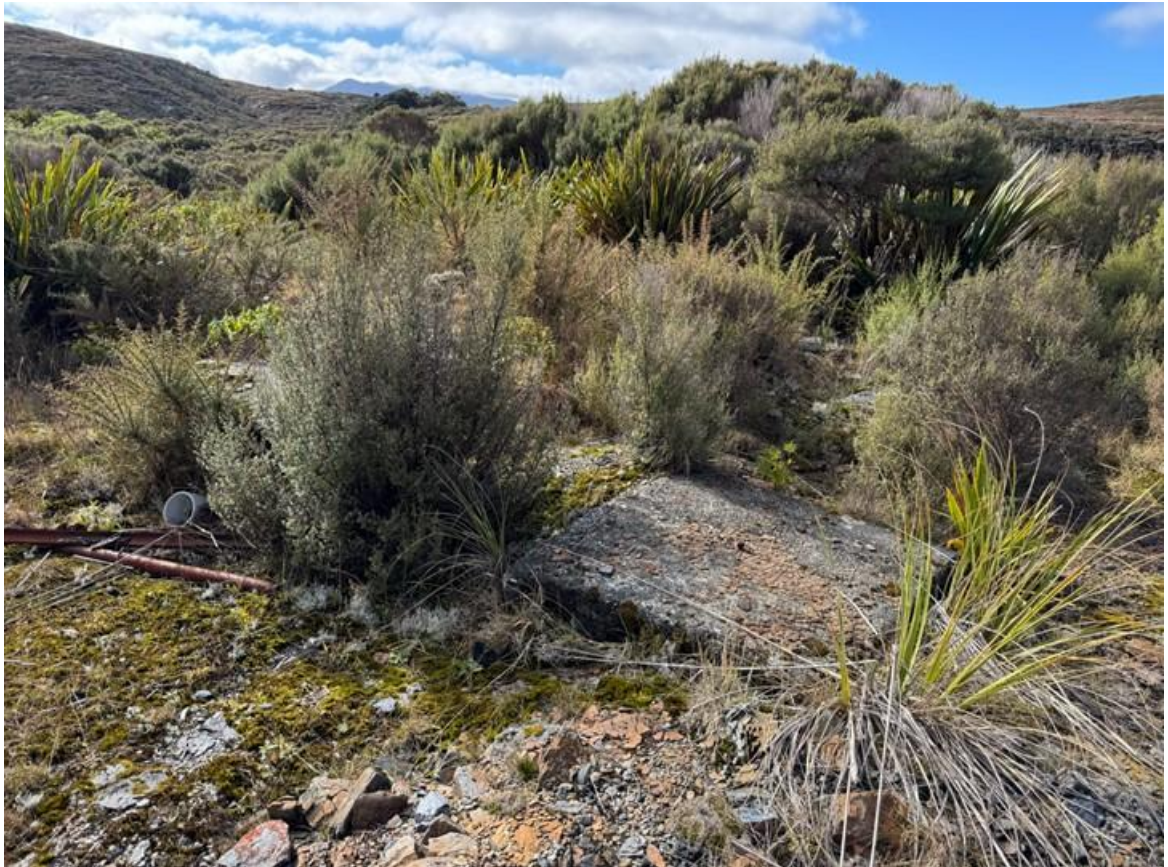
Figure 10. Monocable Aerial Cableway Feature A2 concrete slab foundations beside Whareatea Road that will be removed by the ESE
