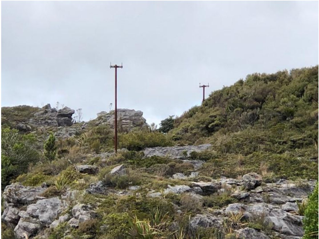
Figure 38. Power poles in the vicinity of the Whareatea Road within the ESE Project sub-area
