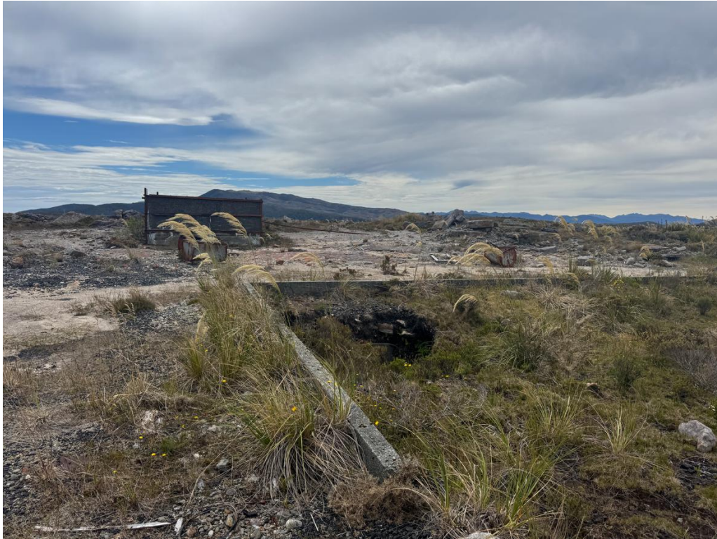
Figure 29. Intact end and side kerbing at Sullivan Mine entrance (Feature 23), showing backfill (right of retaining). The concrete water tank (Feature 34) and some mine boxes or tubs are in the background
