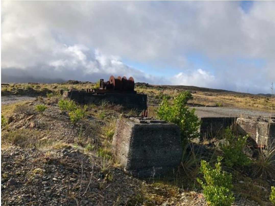
Figure 27. The Sullivan Mine gantry foundations (Feature 25b), winch house foundation (Feature 29) (background) and landing platform (Feature 30)
