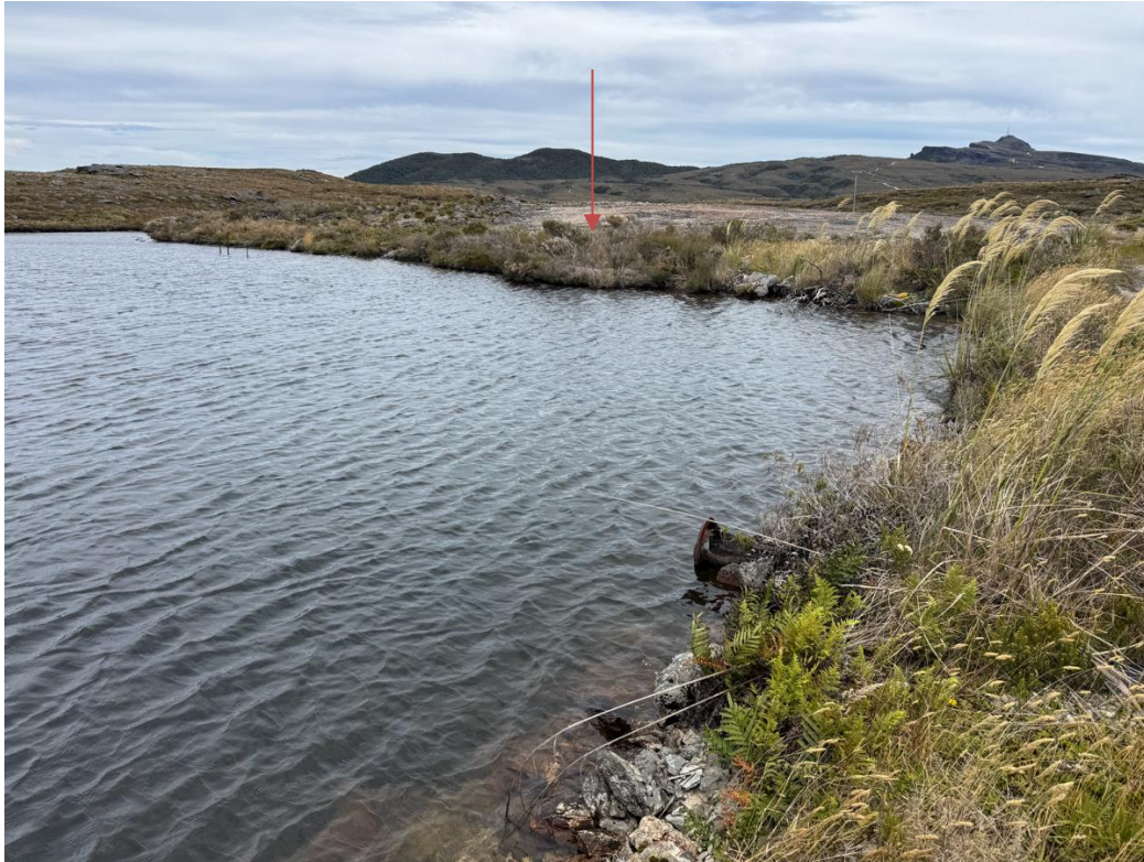
Figure 33. The reservoir at Sullivan Mine (Feature 37) with the pump shed foundation on its edge (arrowed – Feature 38) and metal outlet pipe in the foreground. Fines from one of many Sullivan coal dumps are spread almost to the shore of the reservoir in the background
