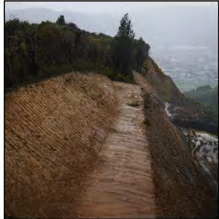
Figure 14. The southern edge of the OBDA, the working face of the quarry.
