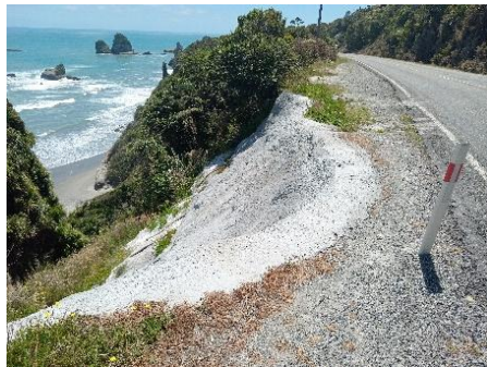
Above left, photo 5: a costly 2023 repair to structural integrity of SH6 edge just north of Waianiwaniwa/ Ten Mile. Note the ongoing impact on the width of the shoulder, leaving a pedestrian, cyclist or motorist nowhere to go if needing to avoid an oncoming or overtaking vehicle.
