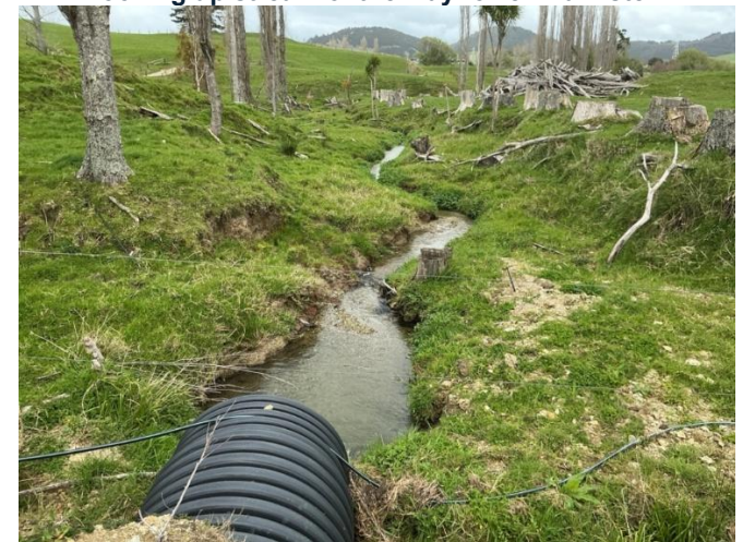
Looking downstream on the Mayflower main stem over a perched culvert.
