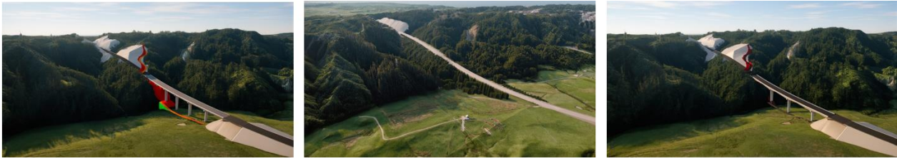
Figure 5: Options assessed as part of the Piroa Stream Crossing alternatives assessment (Option 1 on the left, Option 2 in the centre, and Option 3 on the right). Note that the visualisations present a scenario where vegetation is near or at full maturity).
