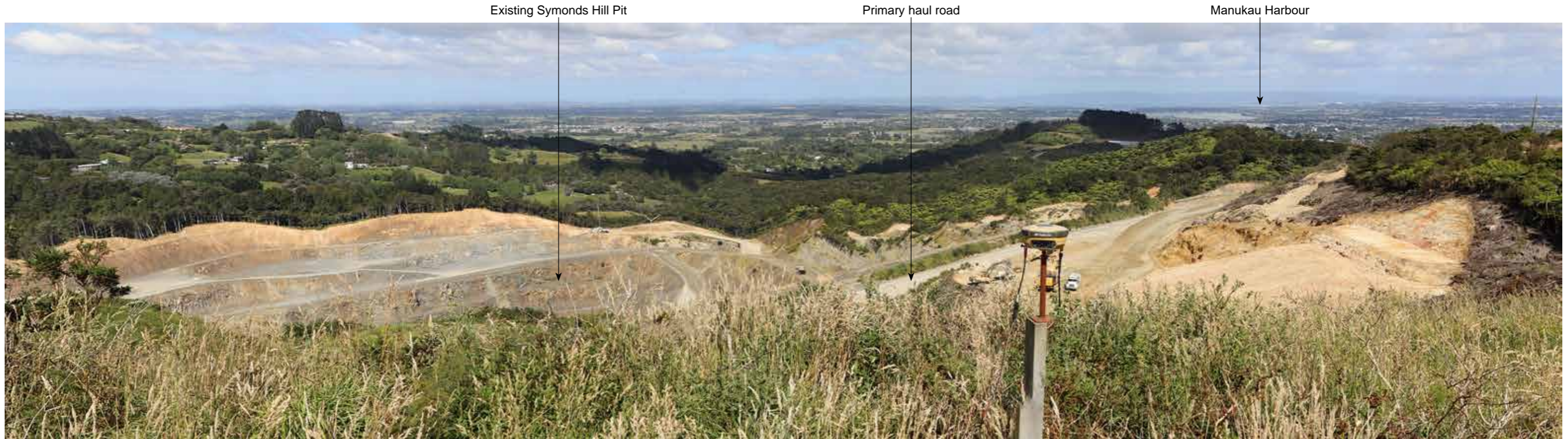
Site Photograph 3 is located on the existing access road, looking in a southwesterly direction.
