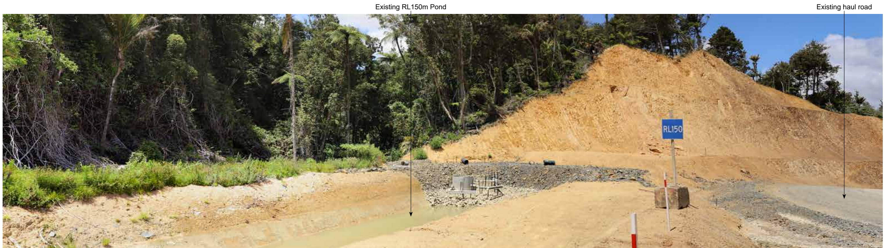
Site Photograph 8 is located south of the existing Symonds Hill Pit on a haul road, looking in a southerly direction.
