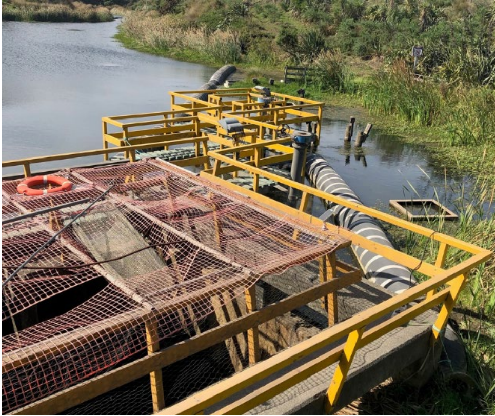
Figure 3: Water Intake Structure Above the Dam on the Wainui Stream
