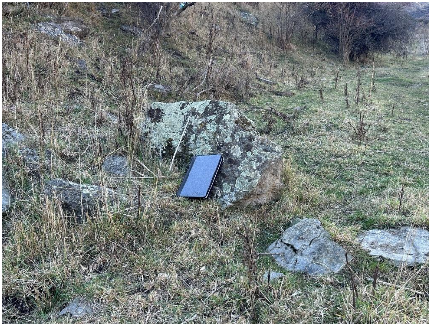
Figure 7: Fallen boulders at the toe of the northern valley slope
