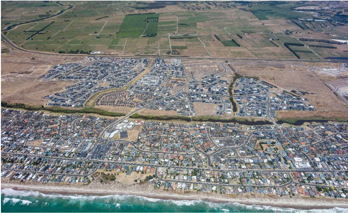
Figure 16 – Oblique Aerial Photography looking south (Source: Bluehaven Group, 2021).
