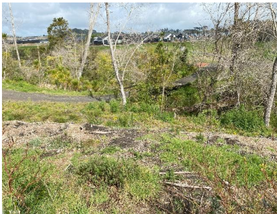
Figure 56. View facing south towards a concrete at timber bridge
