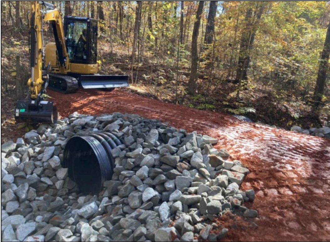
Figure 6: Culvert example (Stantec, 2026b).
