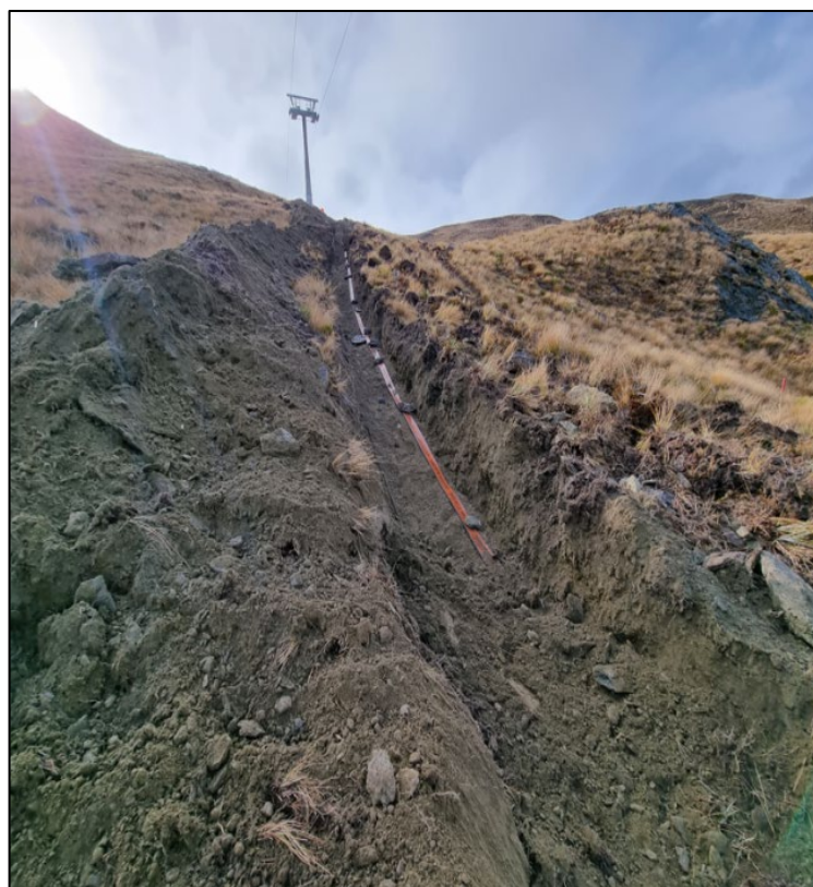
Figure 22: Example of a section of trenching (Source: Enviroscope, 2026).
