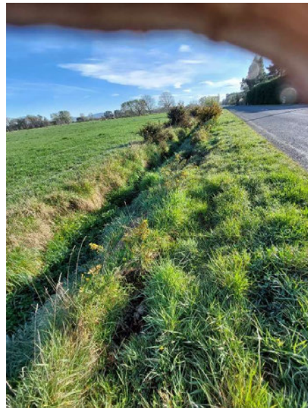
Figure 2. Whites Road drain condition, 29 September 2026, showing narrow rural road with sloping verge to open drain, slumping and low lying land to proposed development site.
