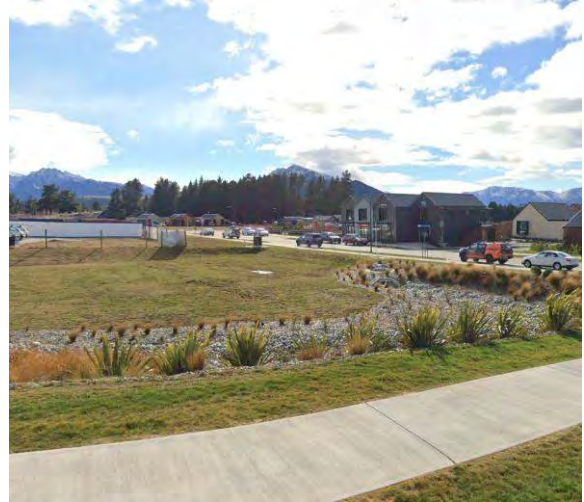
Figure 14B – Example Proposed Dry basin (Northlake, Wanaka)
