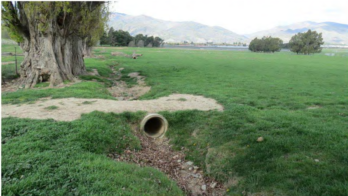
Photo 3511: Water race downstream of western gully outflow. 450mm culvert could block and overtop
