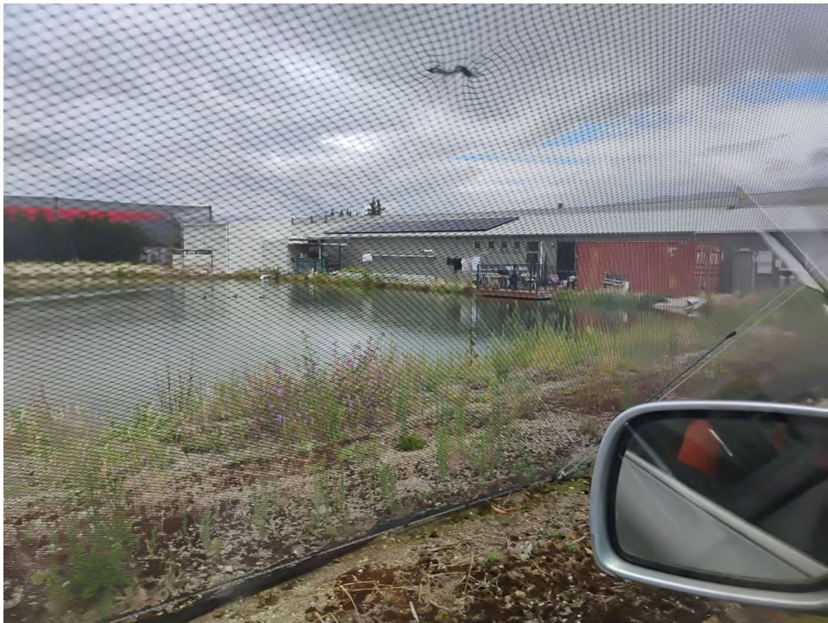
Figure 34: Accommodation, offices and storage sheds
