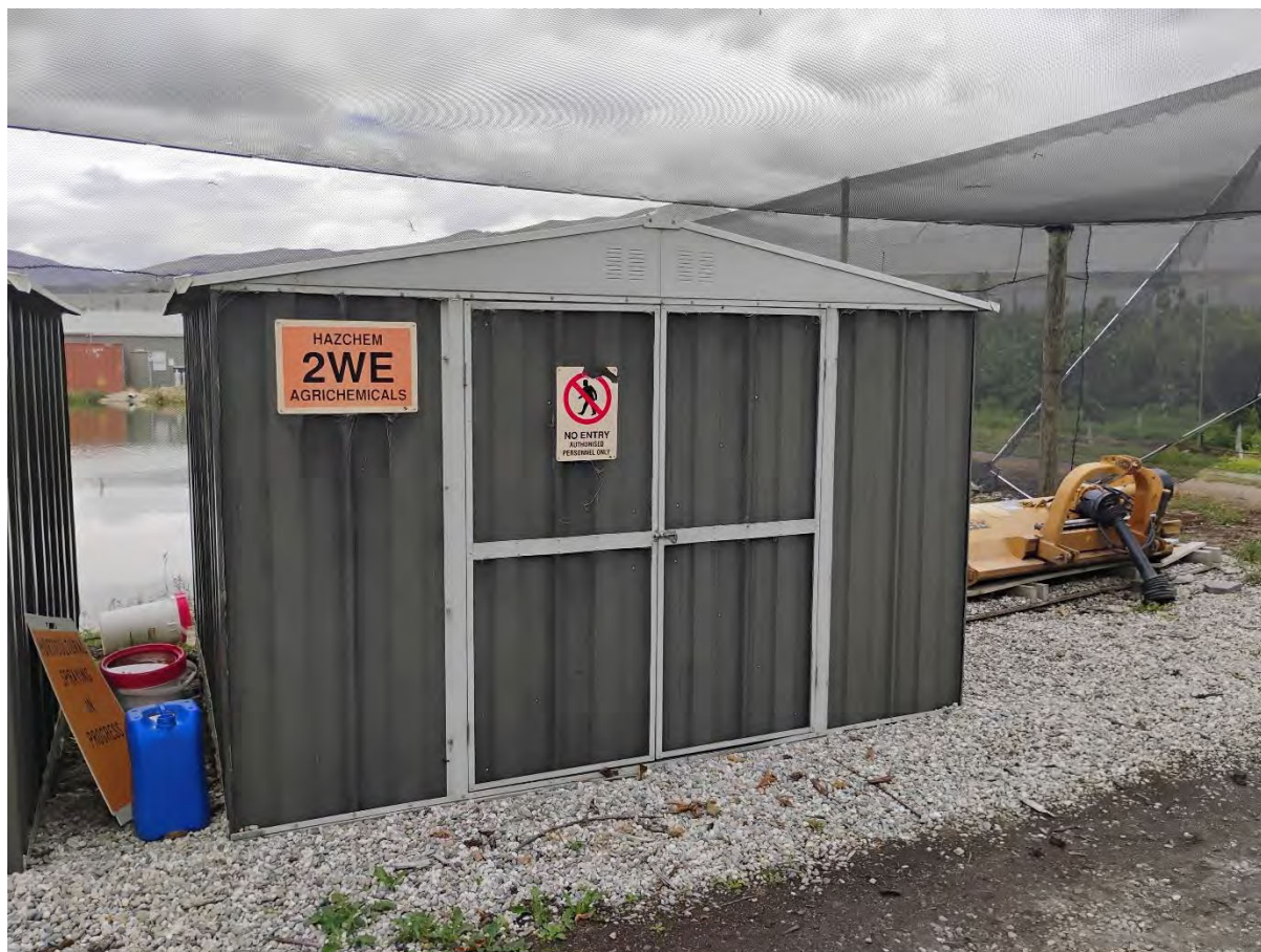
Figure 31: Chemical storage shed
