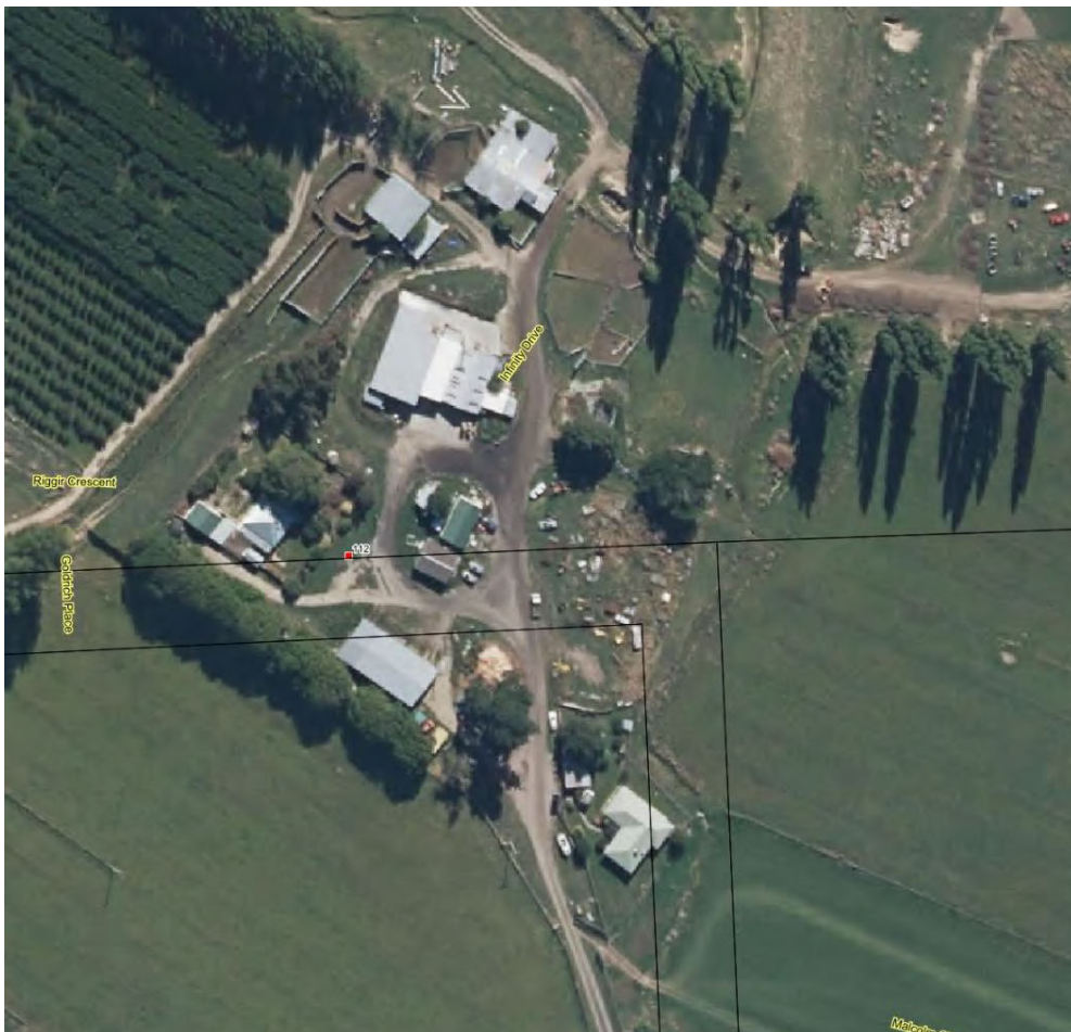
Figure Eight: Aerial photo dated 2019 showing livestock yards and unknown materials storage.
