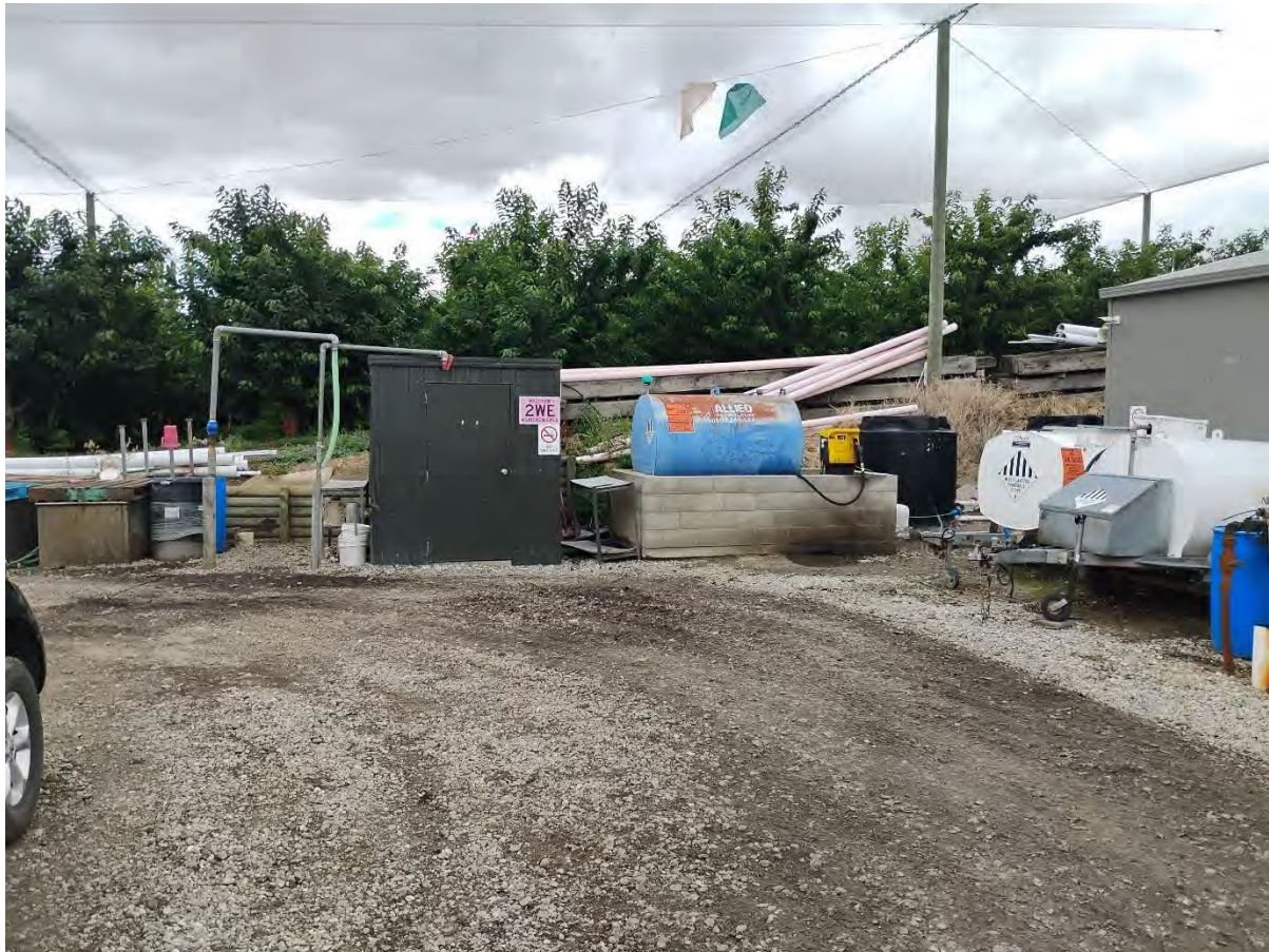
Figure 18: Mixing area, chemical storage shed and above ground diesel tank
