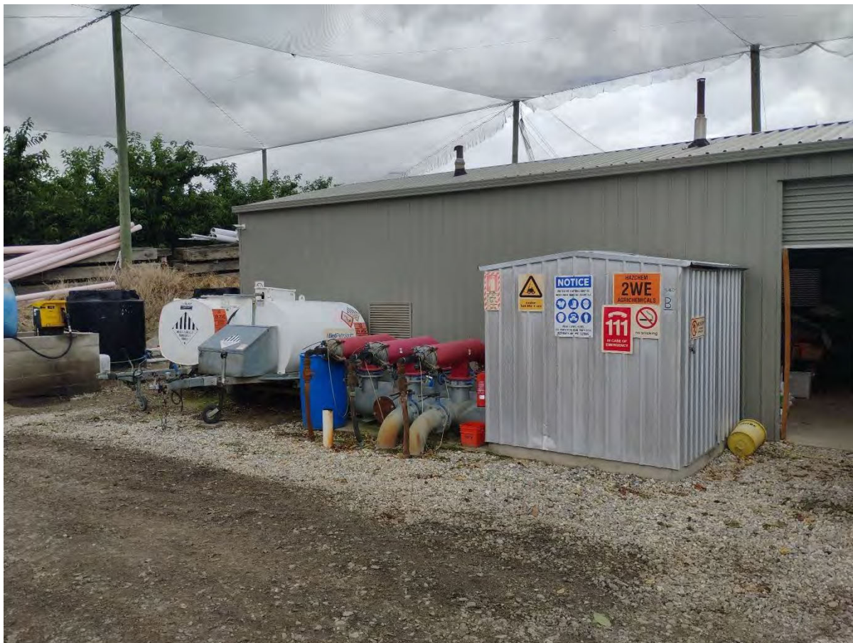
Figure 20: Second chemical storage shed.
