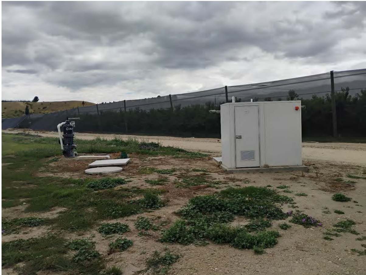
Figure 4: Pump shed near the southern boundary of the site adjacent to the access road.
