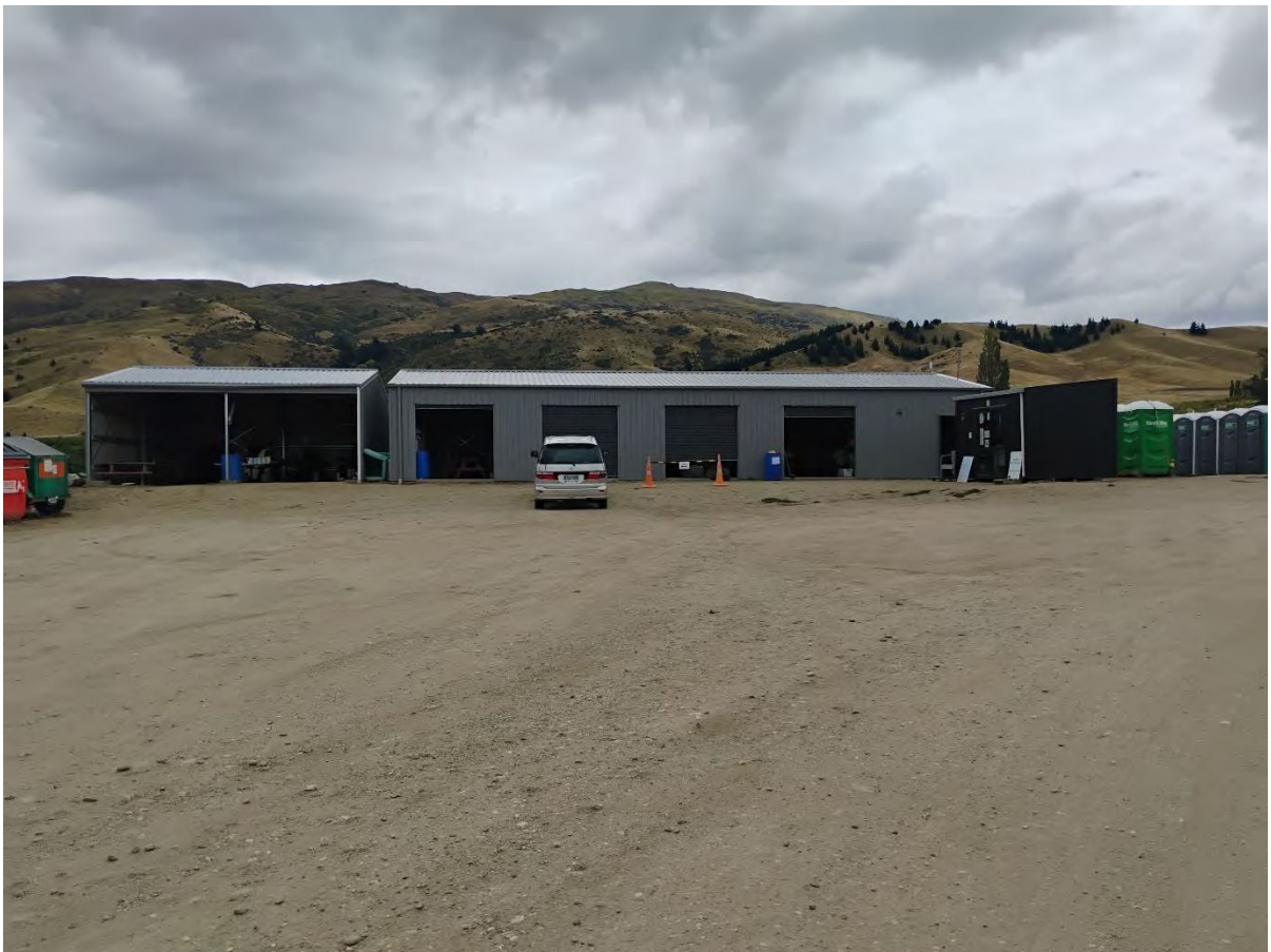
Figure 6: Corrugated iron shed used for storage, cooking and offices
