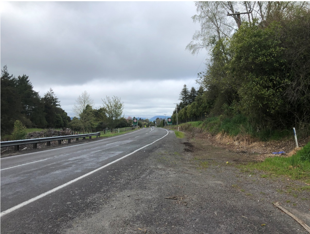
Photograph 2-2: Sh36 / McFetridge Drive sightline south
