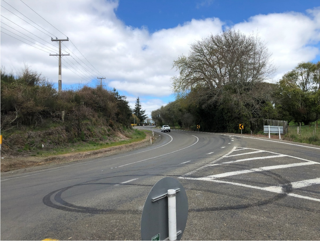
Photograph 2-12: SH36 / Central Road intersection
