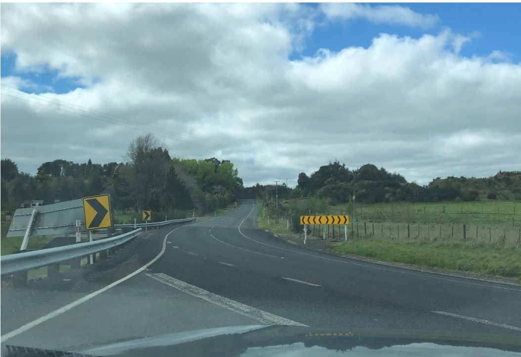
Photograph 2-9: SH36 / Jackson Road Intersection - Sightline North
