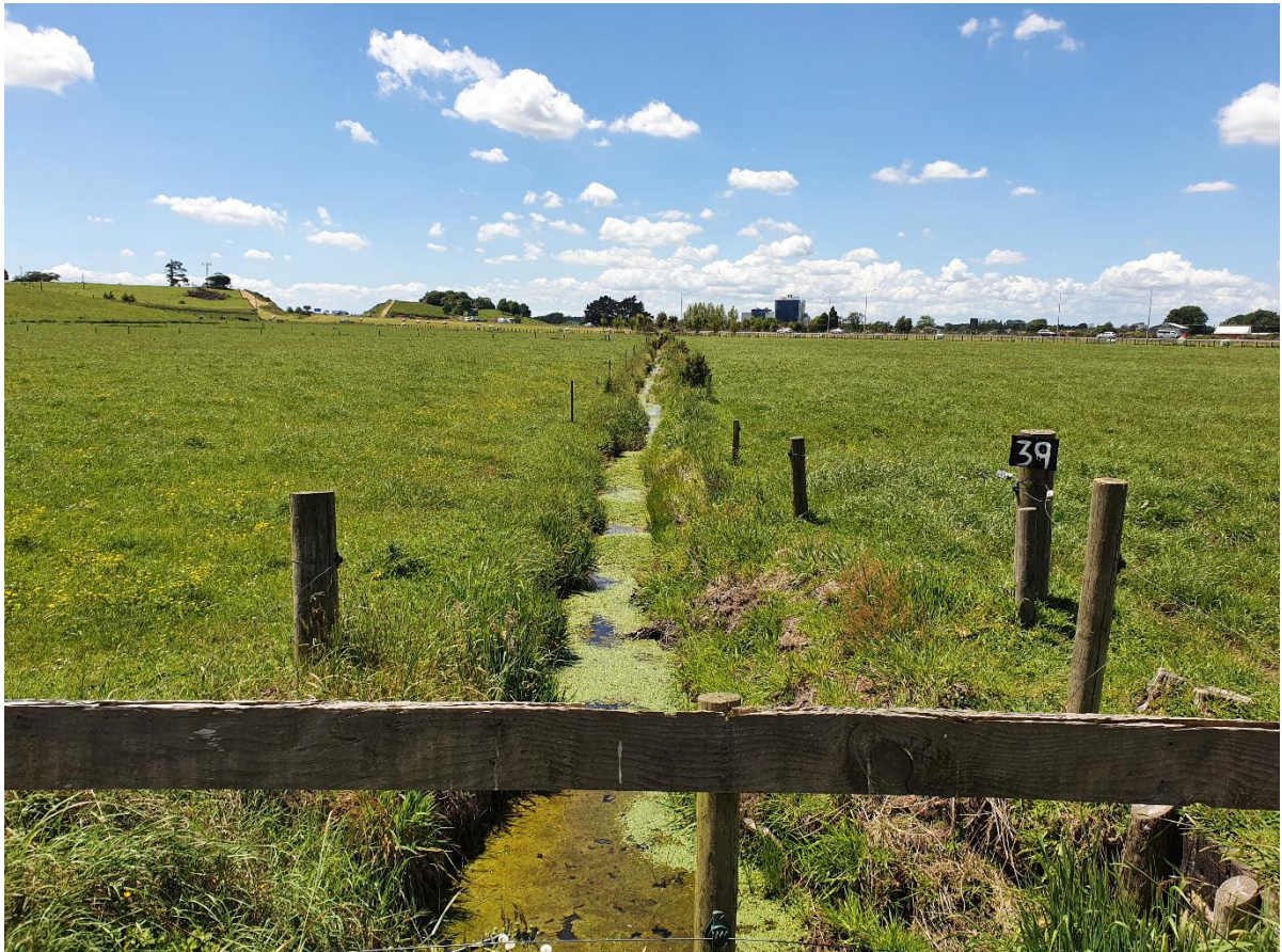
Figure 24: View of Drain M5.
