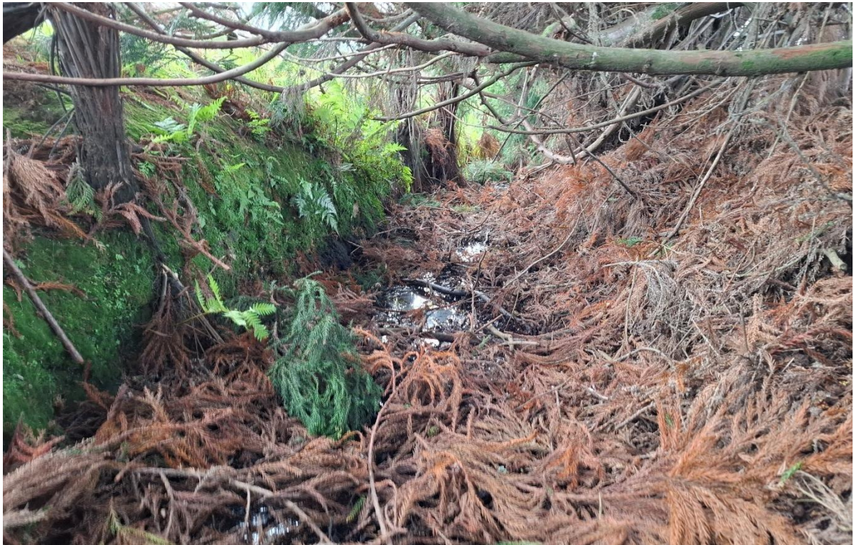
Figure 26: View of Drain M12.
