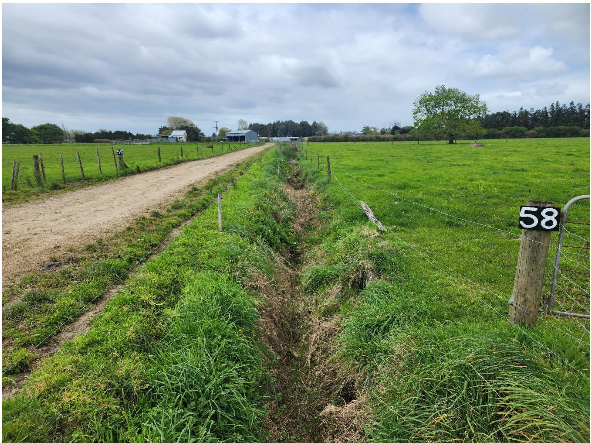
Figure 23: View of Drain M4.
