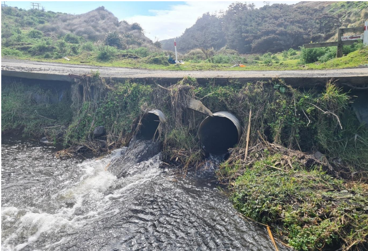
Photo 7: View looking upstream of original culverts, showing hanging culverts and high velocity flow (January 2022).
