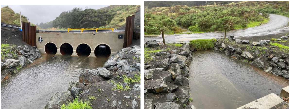
Photo 6: View upstream to newly constructed culverted crossing on Mitiwai Stream (left), and from new crossing downstream to retained crossing (right).
