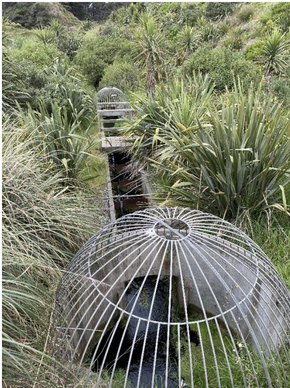
Photo 2: Sections of the fish pass (November 2020).
