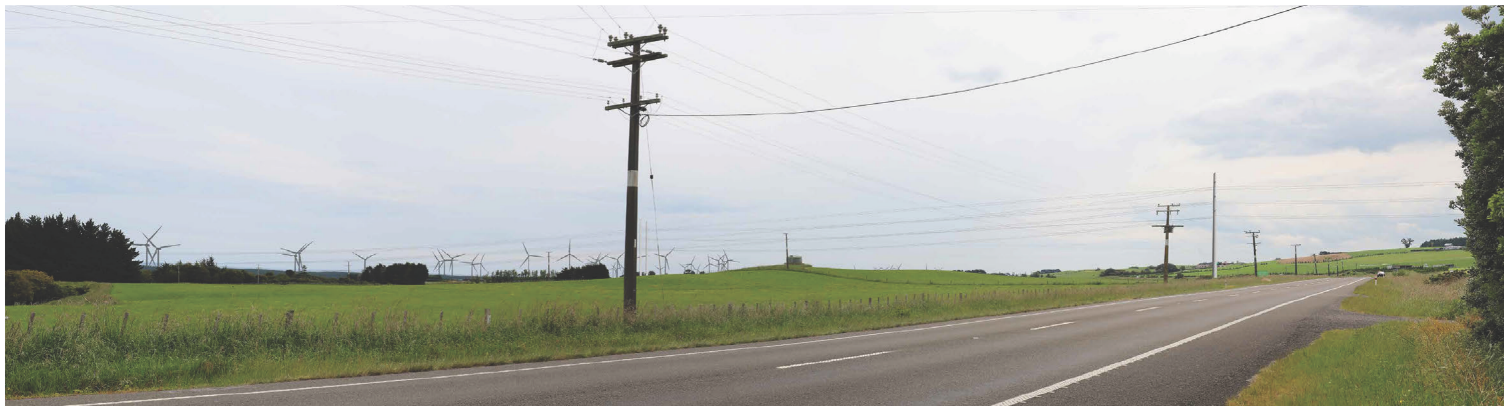
Distance to nearest Waiinu turbine: 3.5 km
