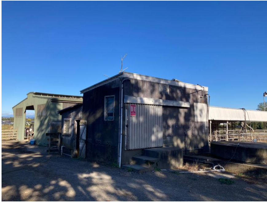
Figure 9: The milking shed. In the approximate area of the 1850s barn.
