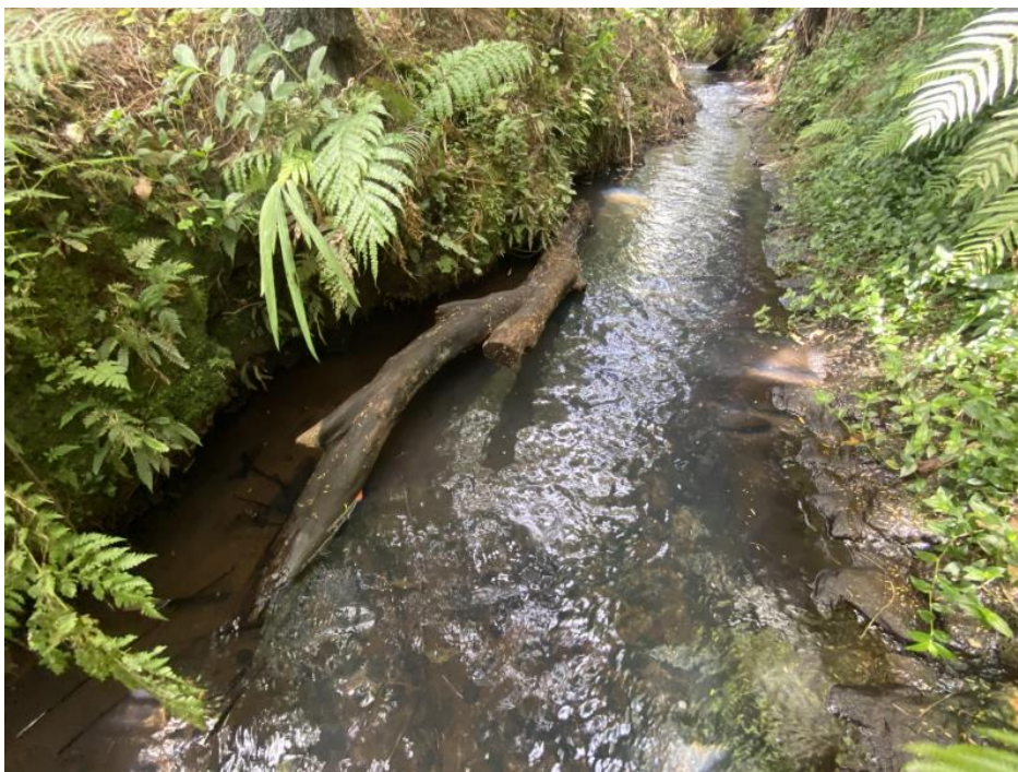
Figure 12: Example of large woody debris to be used in instream habitat construction
