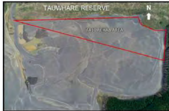
Figure 2.01: TA10 Proposed rehabilitation area
