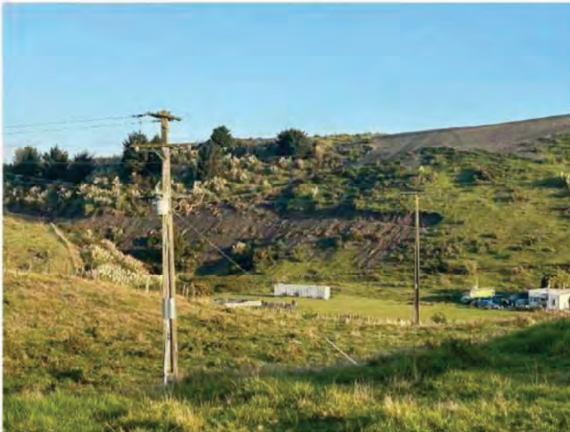
Photo 1: New track cut out for the powerline relocation
