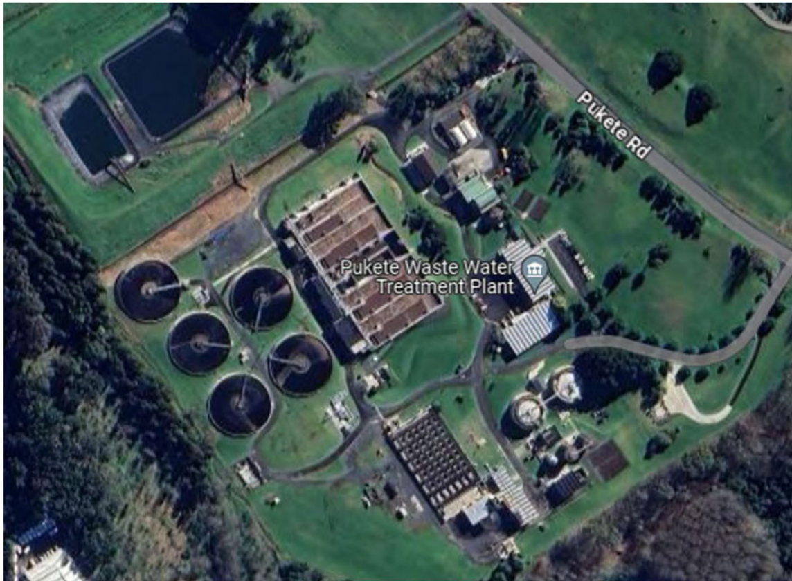
Figure 13 - Pukete Wastewater Treatment Plant (Google Map)
