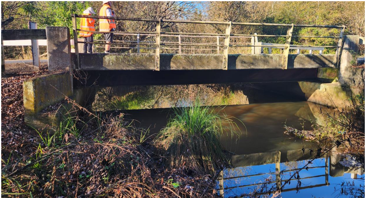
Figure 31 Photo of Crawford Road Bridge
