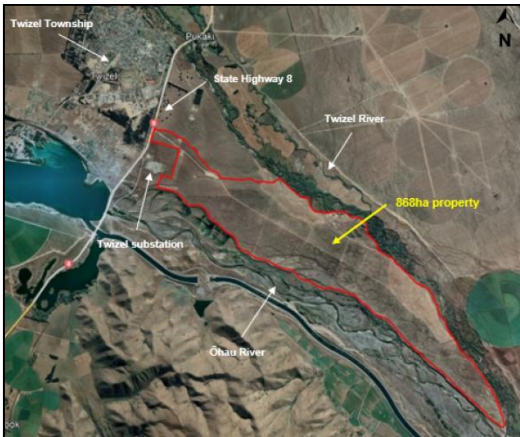
Figure 1.1: Aerial image of the site boundary and the location. Sourced from: Nova Energy Limited.
