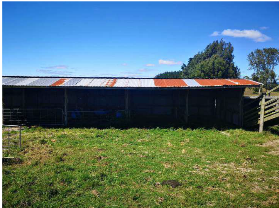
Plate E4: Looking south towards the calf rearing shed.
