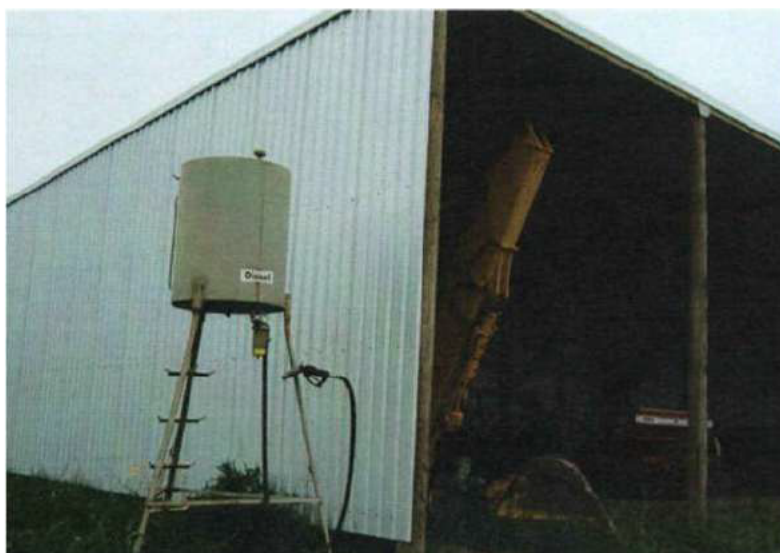
Plate 1: Diesel AST located on south side of eastern implement shed, c. 2010. Image sourced from BC 63962.
