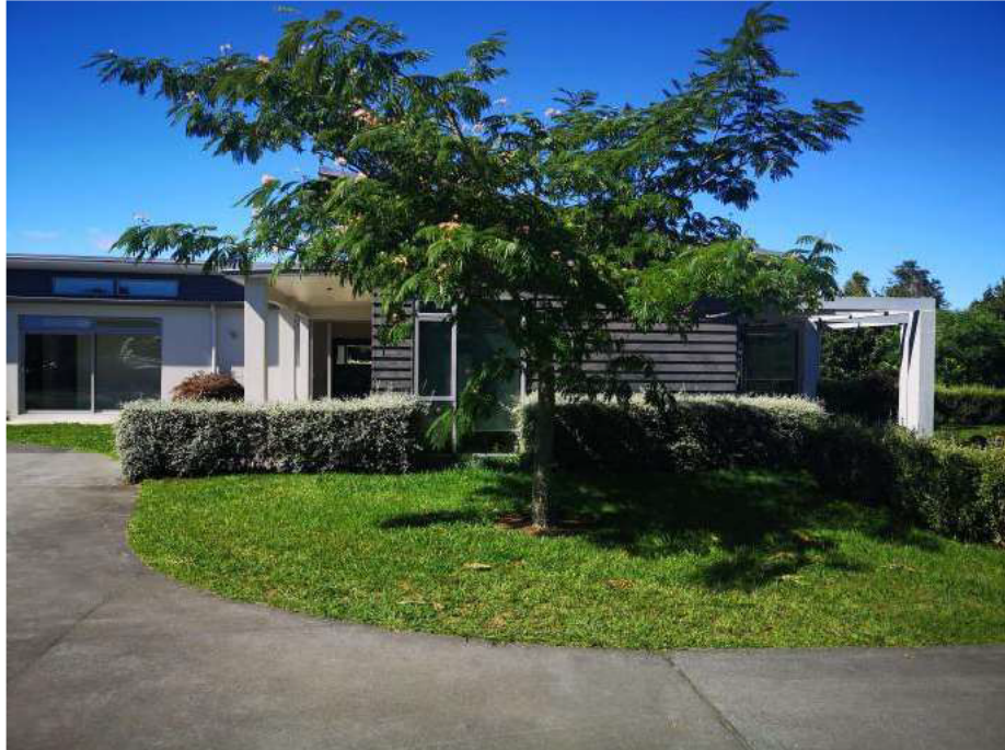
Plate E1: Looking south towards the Milsom family residence.
