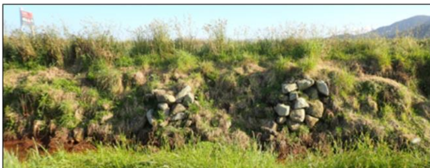
Figure 17: POI 003 Stacked drystone structure beneath Cargill Road (Wooller, 2024).
